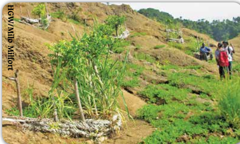
Ledges of earth and dried grass built on a deforested hillside in the Petit-Goâve region. Peanut plants can be seen encroaching in the lower right.
