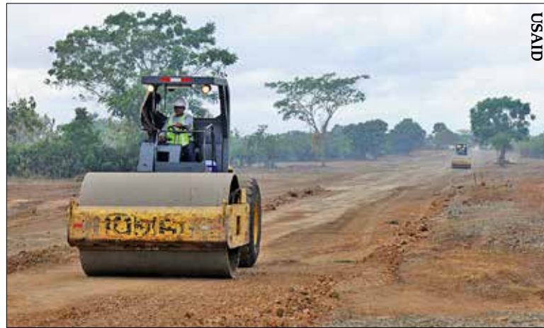
...steam rollers clear road into the 600 acre industrial park.
