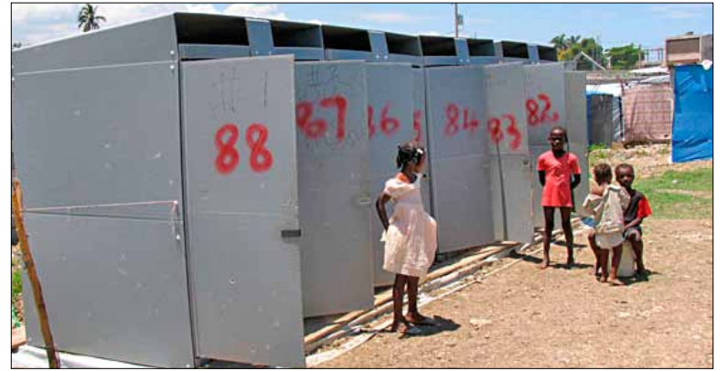
Out of 12,000 latrines needed in the IDP camps, only 4,579 (38%) were functional. Many desludging activities (cleaning of latrines) ceased at the end of August for lack of funding
